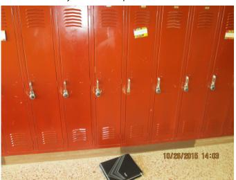
The corridors have mostly terrazzo floor and are in fair to good condition. However, the second floor have 8"x8" vinyl asbestos tiles located on the south, east and wet corridors which are in fair condition.
