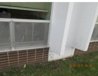
The main entrance canopy and south canopies are constructed with painted precast panels. The soffit paint is peeling and stained in some areas. The lenses on some of the light fixture area discolored.
